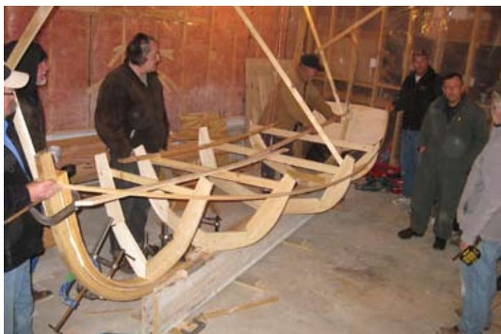
Battening the shape of the boat with five molds
